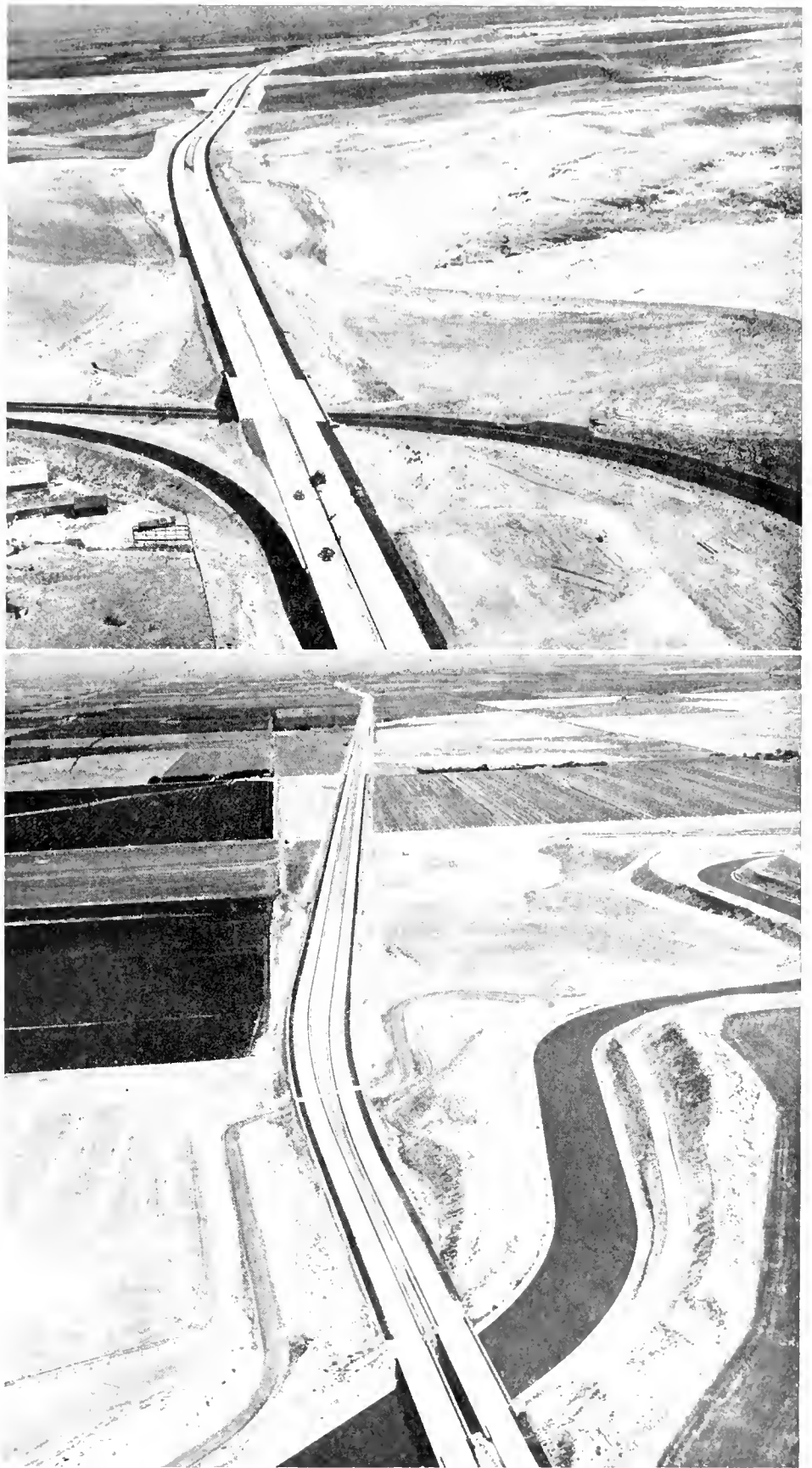
New Altamont-Tracy Expressway. UPPER: Mountain House interchange looking east. LOWER: Expressway crosses Delta-Mendota Canal, an right.
